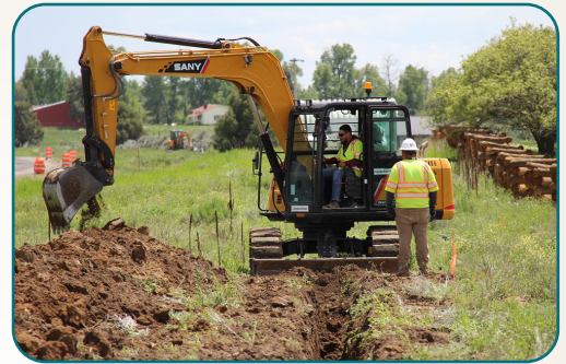
Crews excavate a trench along U.S. 84 south of Chama.
